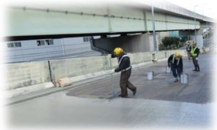
Waterproofing of bridge concrete slab
