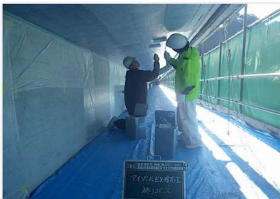
Concrete surface coating method
