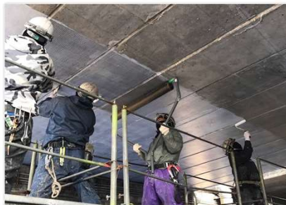
Prevents peeling-off of concrete
