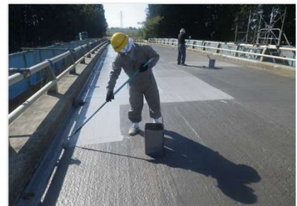
Waterproofing of bridge concrete slab
